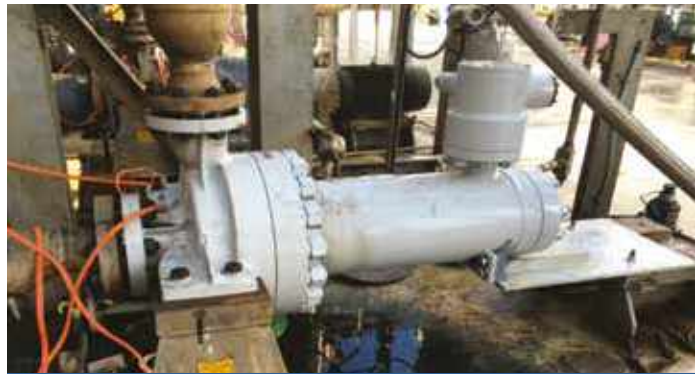
Pumping a Caustic Solution. Our canned motor pump eliminated a seal leak that was occurring every 3 months.
