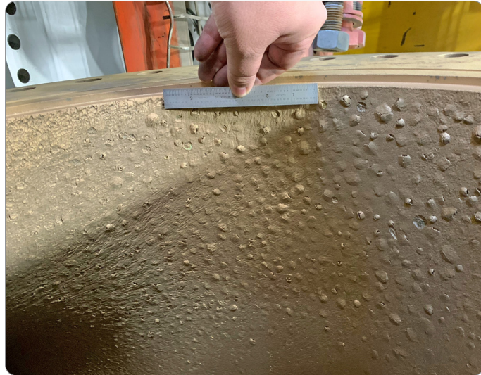
Image 3: Corrosion on the internal surface of discharge elbow.
