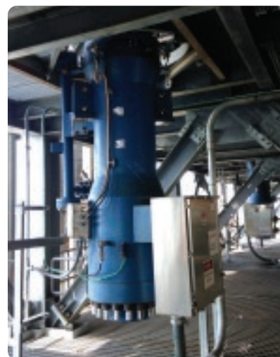
Radiant Syngas Cooling circulating pumps installed in Edwardsport, IN
